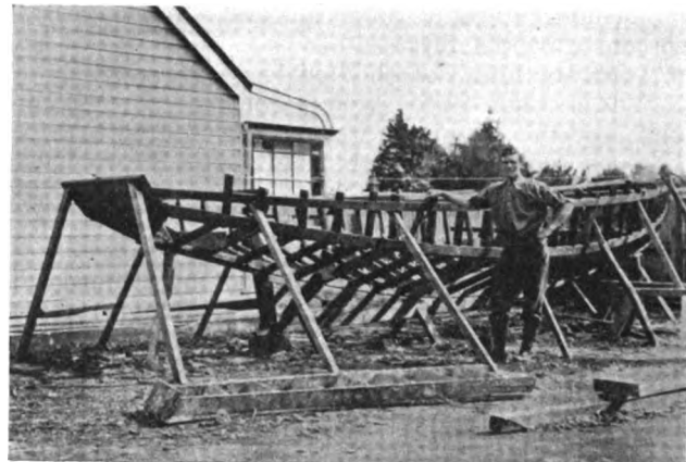
Sea Bird. Building at Christchurch, N. Z., by Mr. J. F. Day
